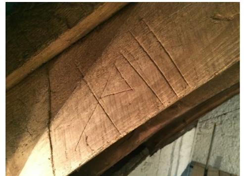
trusses slot together, having been made on the ground and hauled up to the roof in pieces, ready for assembly.
